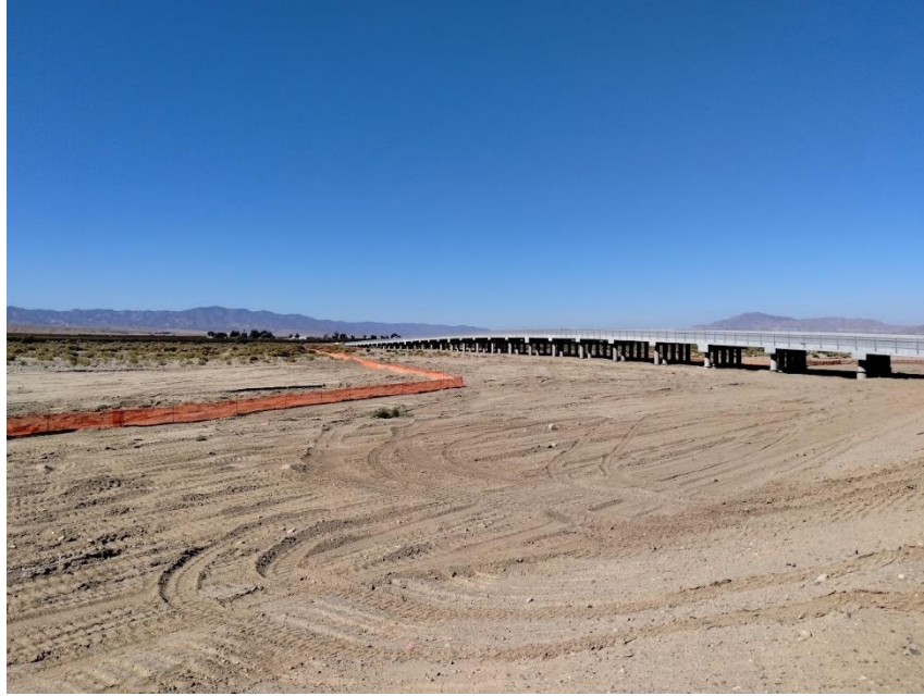
Figure 2 Foothill Road Bridge over Cuyama River project Bridge No. 00L0047 AFTER
