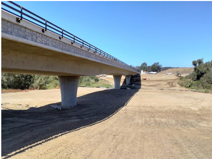
Figure 3 Bridge No. 51C0006 Floradale Ave Bridge over Santa Ynez River AFTER
