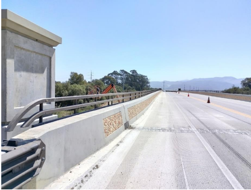
Figure 4 Bridge No. 51C0006 Floradale Ave Bridge deck
