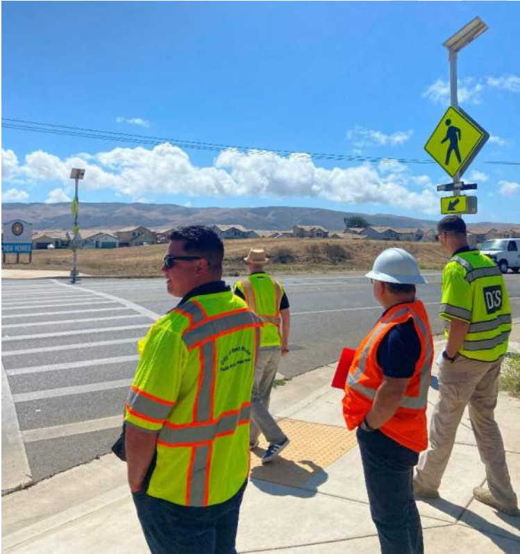
FIGURE 14. SR 166 AND OBISPO STREET SOUTHWEST CROSSWALK
