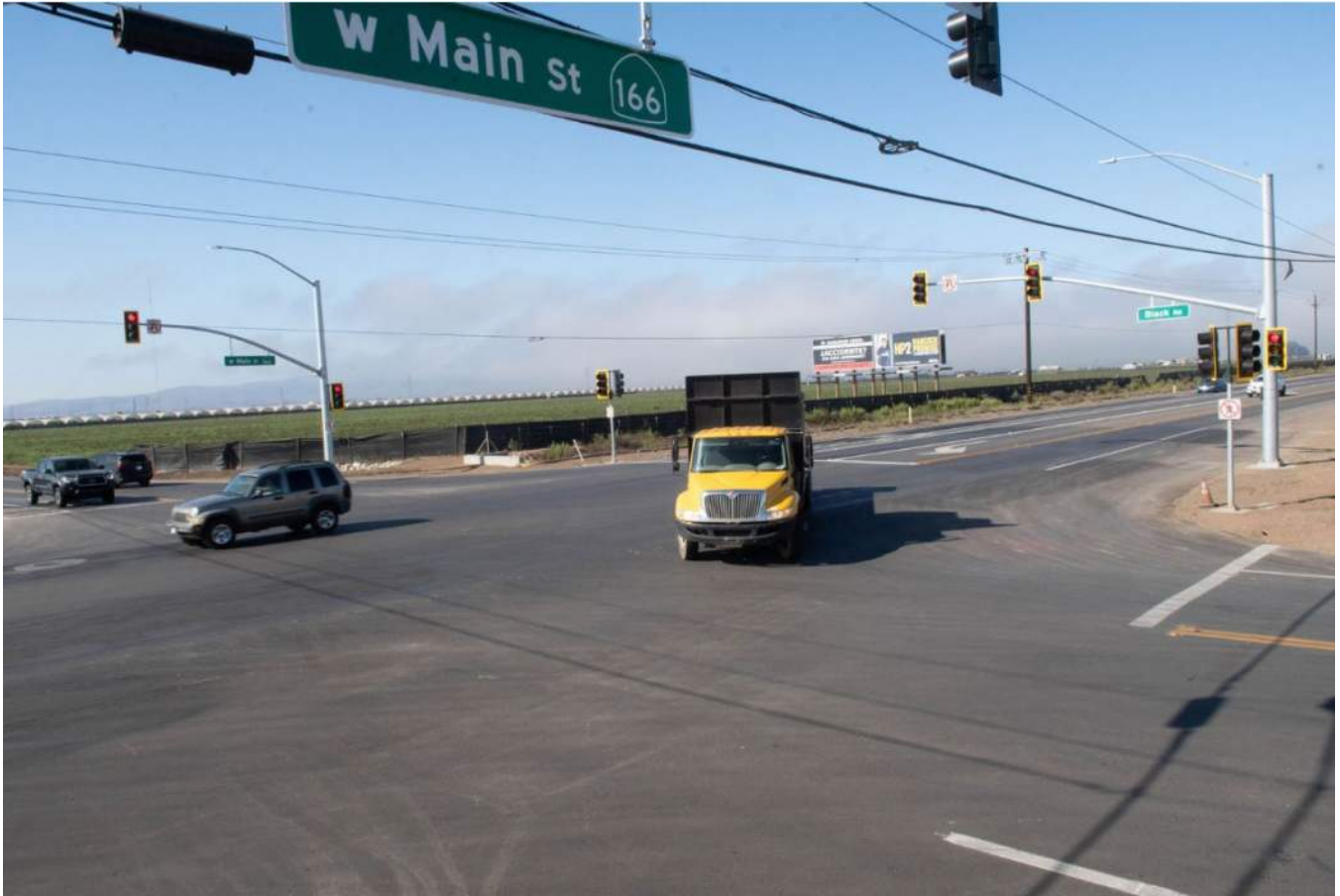
FIGURE 3. SR 166 AND BLACK ROAD TRAFFIC SIGNAL CONSTRUCTION COMPLETION (SOURCE: SBCAG SR 166 AND BLACK ROAD RIBBON CUTTING)
