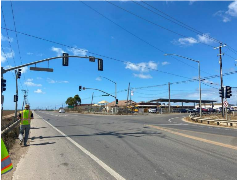
FIGURE 18. SR 166 AND BONITA SCHOOL ROAD EXISTING CONFIGURATION - SOUTHEAST CORNER
