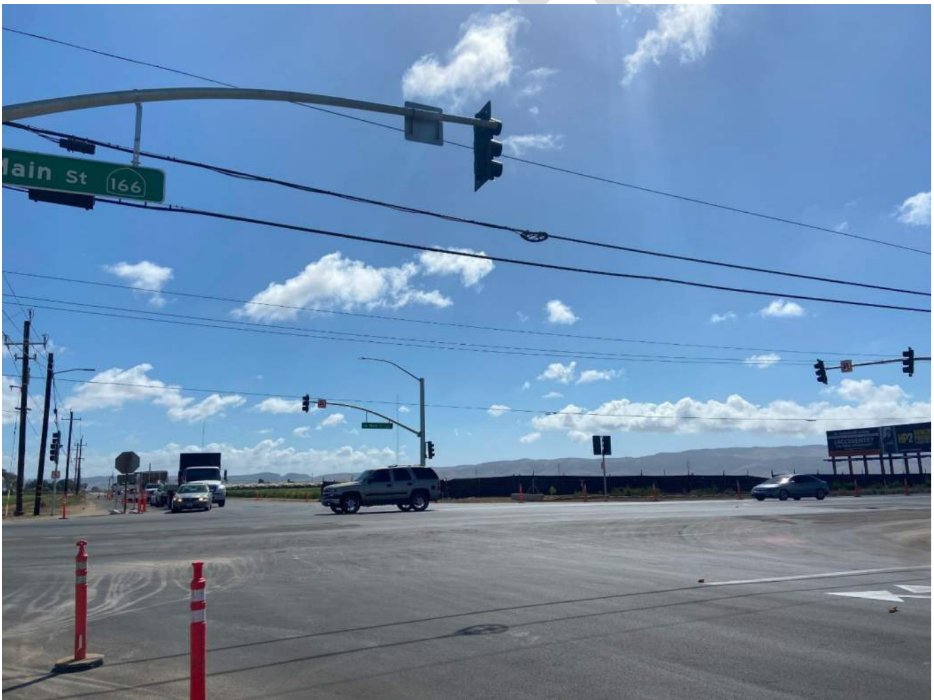
FIGURE 23. SR 166 AND BLACK ROAD EXISTING CONSTRUCTION - NORTHEAST CORNER
