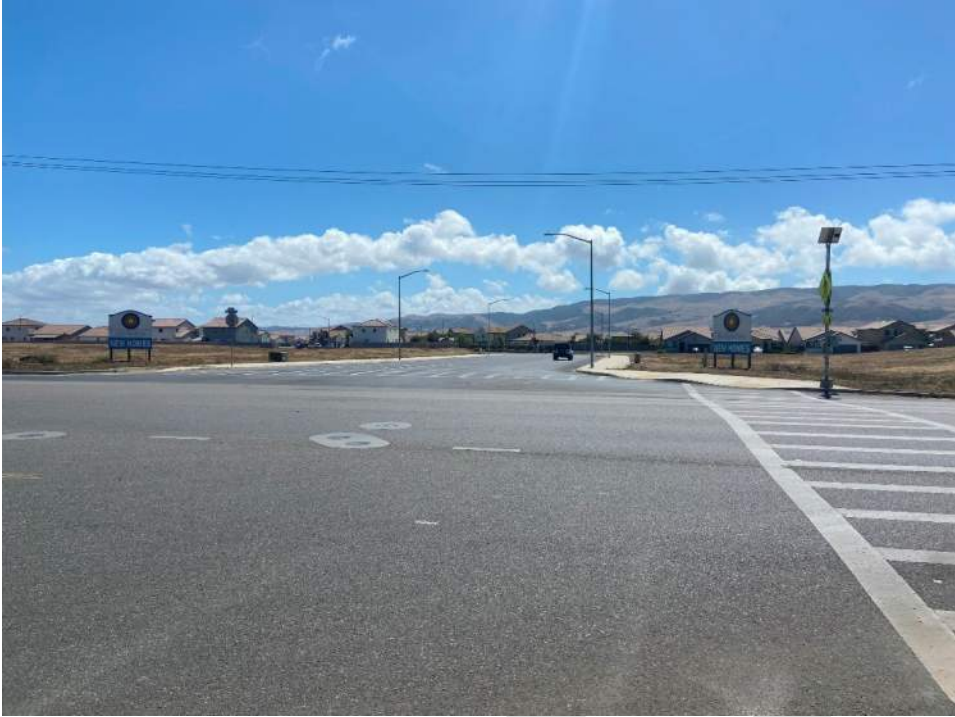
FIGURE 13. SR 166 AND OBISPO STREET SOUTHWEST CORNER – CROSSWALKS
