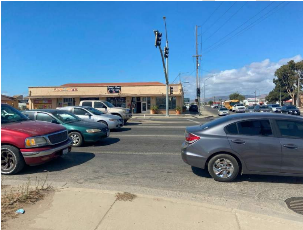
FIGURE 25. SR 166 AND BLOSSER ROAD APPROACH - SOUTHWEST CORNER
